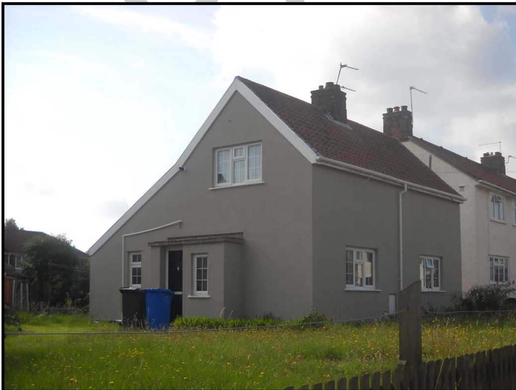
Photograph - Property after external wall insulation was installed, SAP rating Band C
