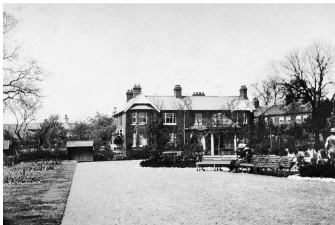
Sewell Park, north end looking west
