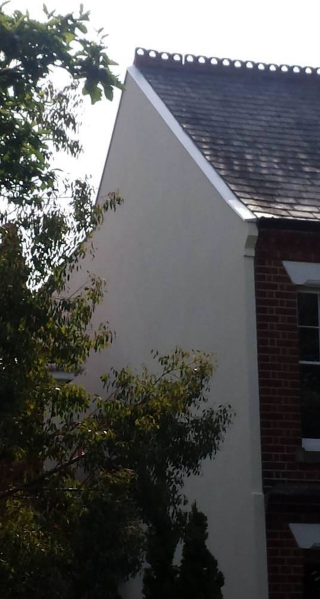
Elevation showing eaves, flashing and capping
