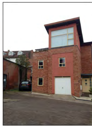
EXISTING SOUTH VIEW LOOKING NORTH
