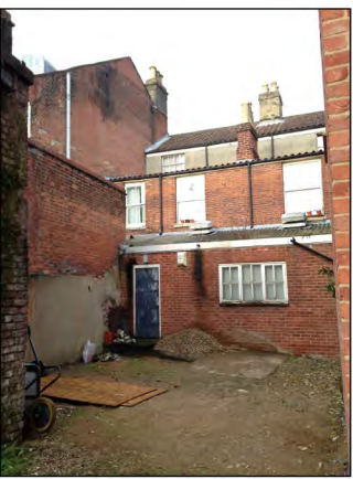
EXISTING NORTH-WEST VIEW LOOKING NORTH
