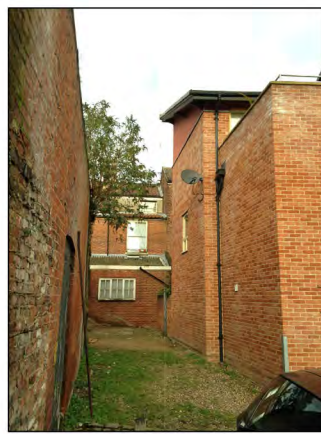
EXISTING SOUTH-EAST VIEW LOOKING NORTH
