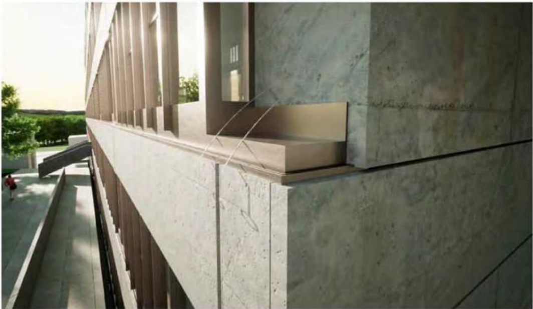
Fig 6.43 CGI of existing cill detail
