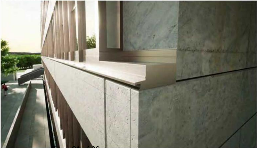
Fig 6.44 CGI of proposed cill detail
