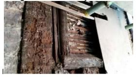
Initial dismay about the temporary closure of one of our main display rooms for ceiling repairs following leaks was mitigated by the promise from NORSE of carrying out some long-needed additional work on a gable in the Coach-house courtyard. But what should have been a simple repair however, turned into a major headache when it was discovered that the timbers in that part of the building had been severely affected by wood-boring beetle.
