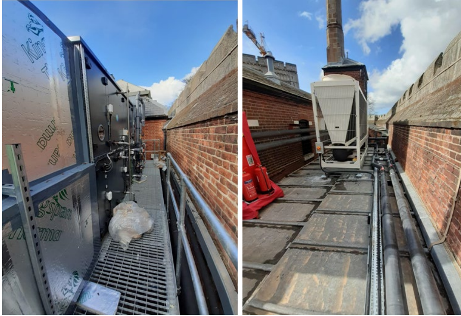
New air handling and chiller plant installed at roof level
