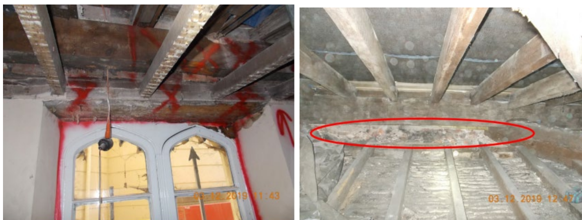
Areas of dry rot marked up on site & affected structural timbers highlighted in the roofspace
