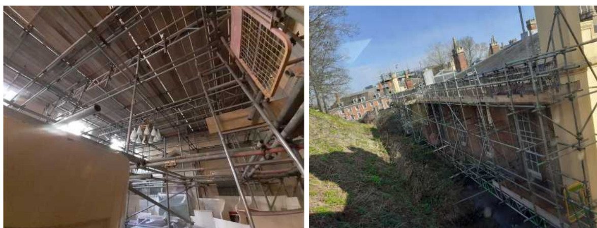
Interior bird nest scaffolding and external elevation scaffolding to allow contractor access
