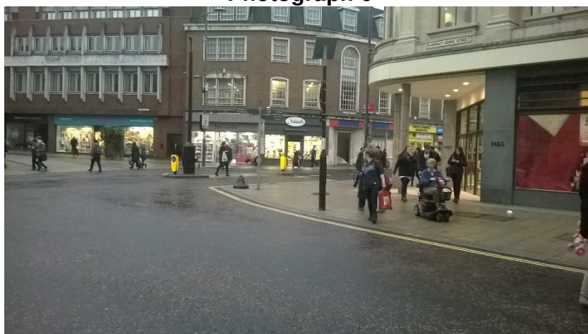
Pedestrians preparing to cross at location B. Note raised table surfaced in asphalt with chippings.
