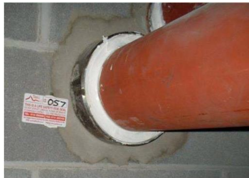
New pipe fitted with intumescent collar
