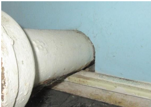
Waste pipe with no intumescent collar
