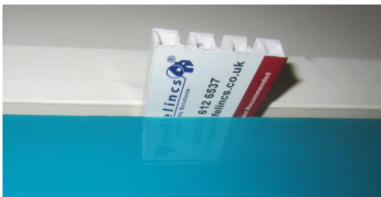
Gap between door and frame exceeding 4 mm recommended tolerance
