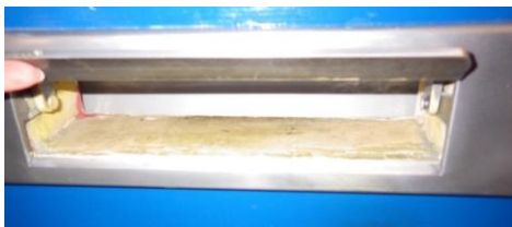
Example of letter flap with no intumescent liner
