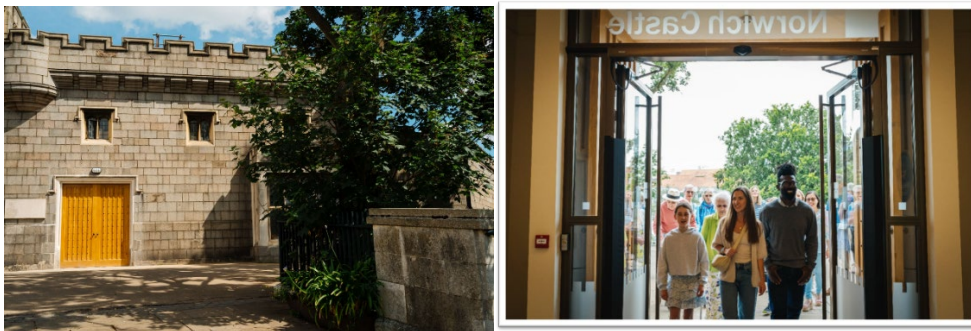
New visitor entrance at Norwich Castle
