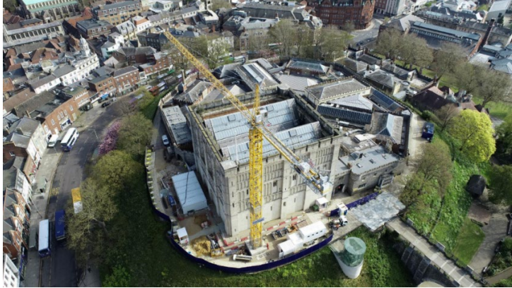
Drone image of the construction site
