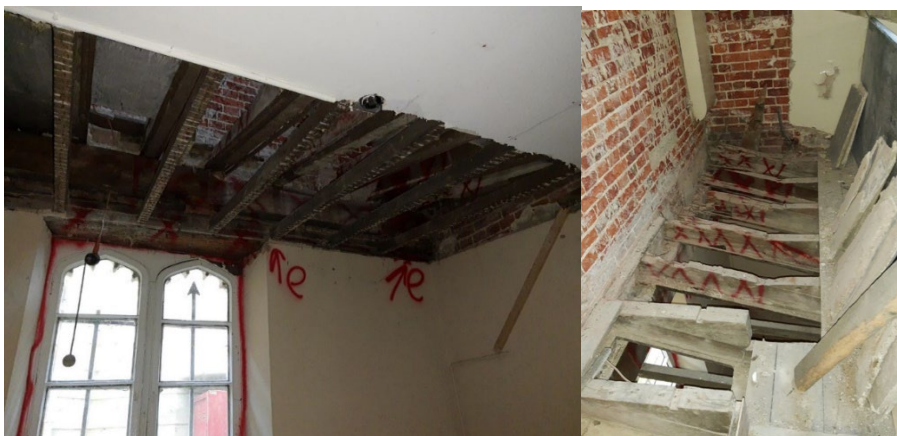
The SW corner of the Courtroom and details of affected structural timbers
