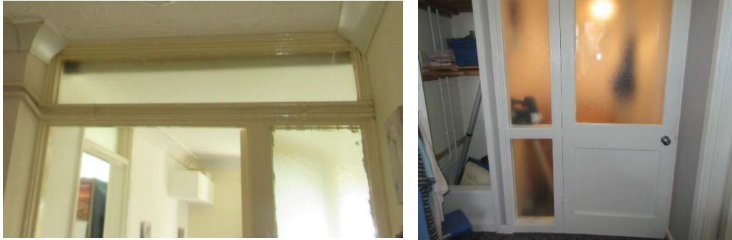
Two examples of non-fire rated visual panels to door and side panel.
