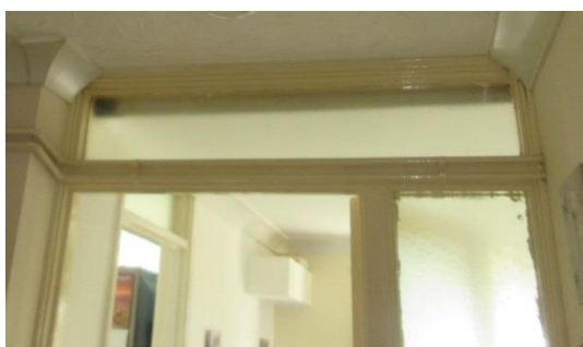
Non fire-rated visual panels to door and side panel
