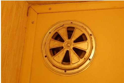
Ventilation duct with no intumescent liner
