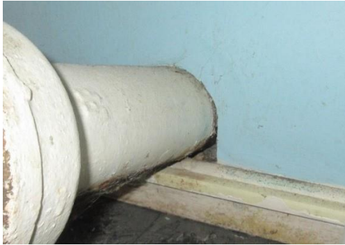
Waste pipe from WC penetrating compartment panel
