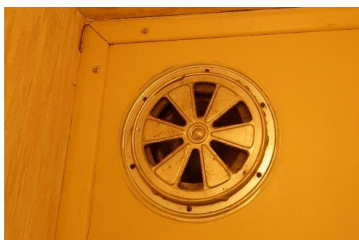
Variety of ventilation ducts with no intumescent liner
