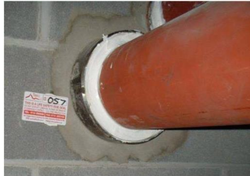
New pipework fitted with intumescent collar
