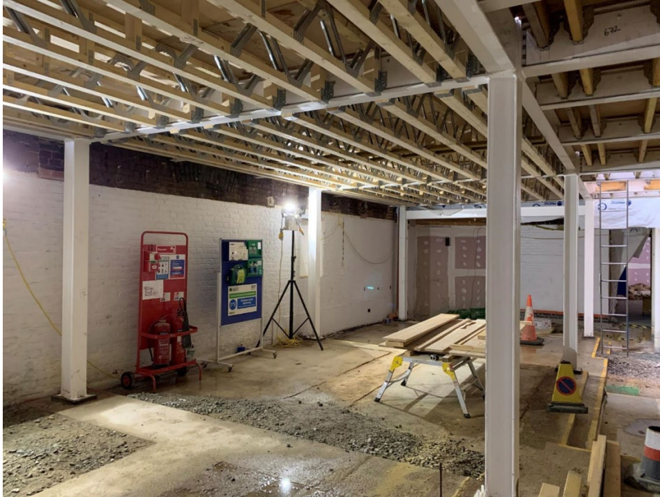
New steelwork and floors in the new WC block area
