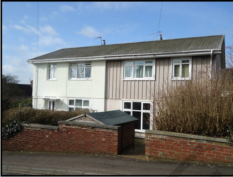
Right to left – before and after EWI has been installed on BISF homes
