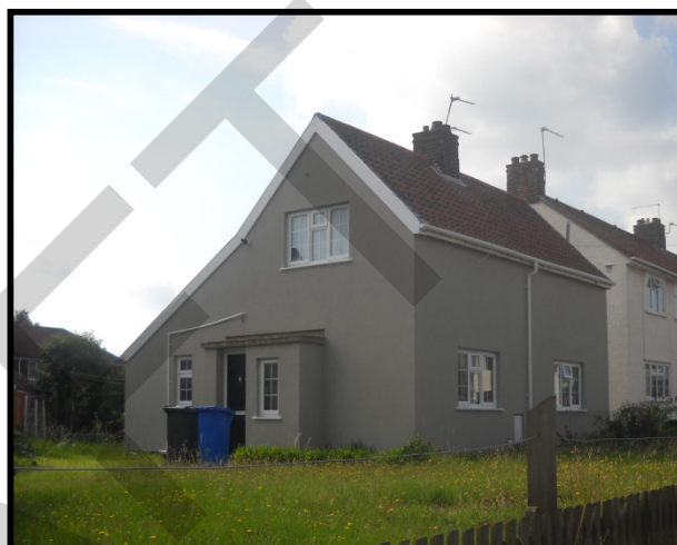
Property after external wall insulation was installed, SAP rating Band C
