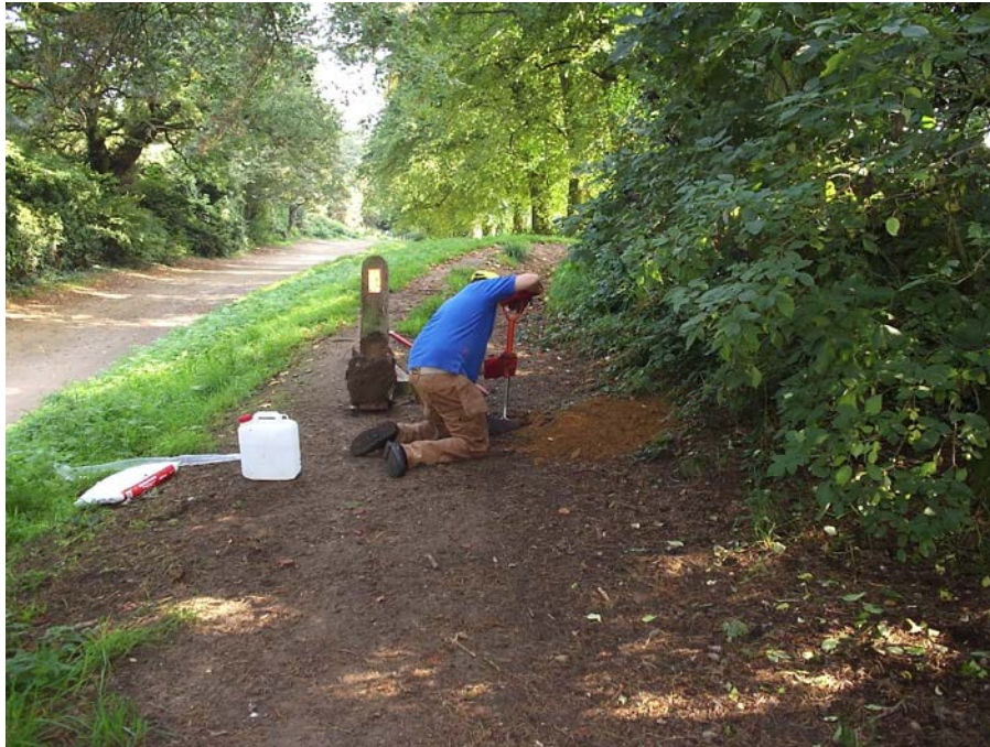
Bollard installation to prevent vehicle access onto Gilman Open Space
