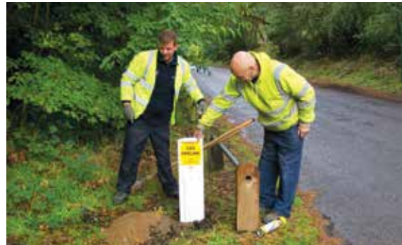
Gas pipe line marker installation by National Grid
