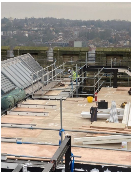
Installation of rooftop platforms on Keep
