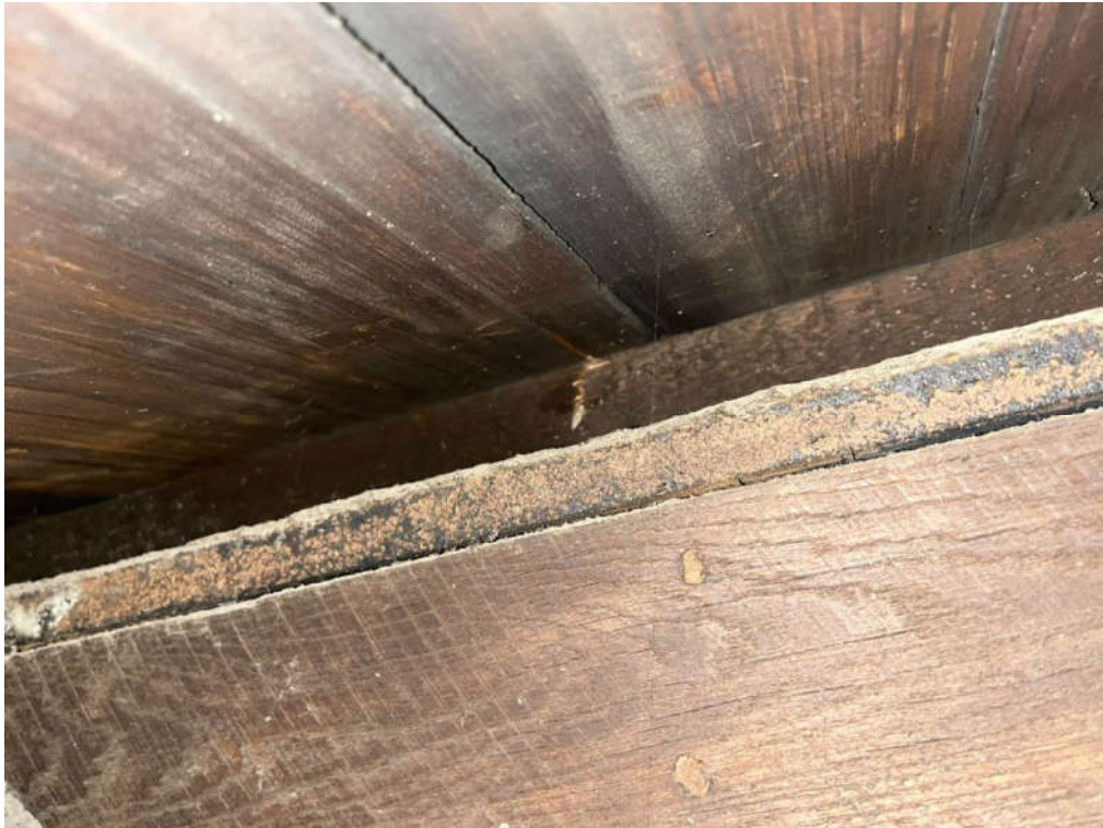
Photograph 43 – Top flange of steel rafter showing signs of rust
