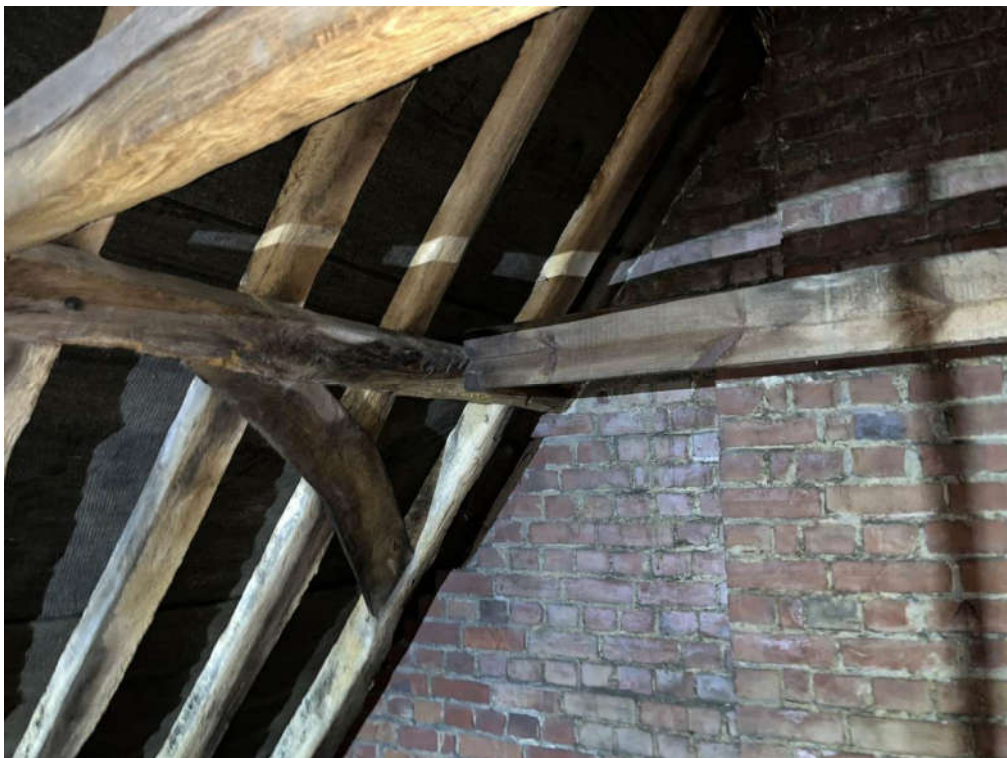
Photograph 70 – Roof structure dry where entering East gable
