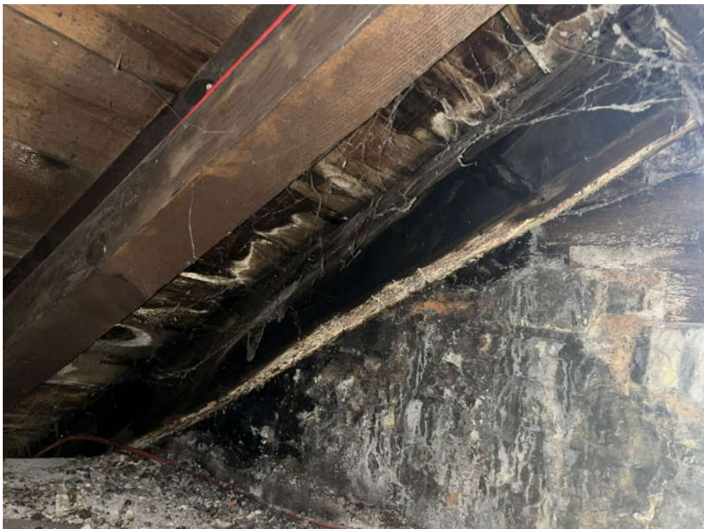
Photograph 32 – Damp common rafter against North Wall in organ loft
