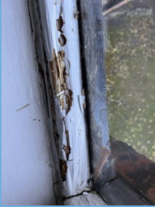
Cloister window at end of life
