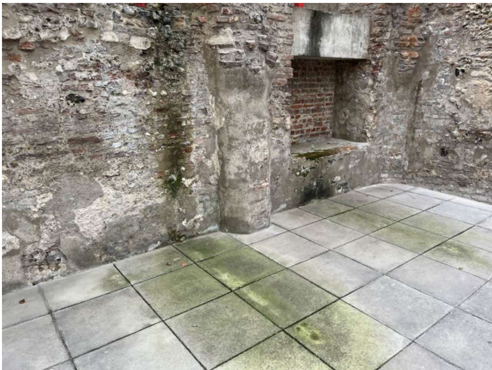
Photograph 94 – Signs of water ingress
