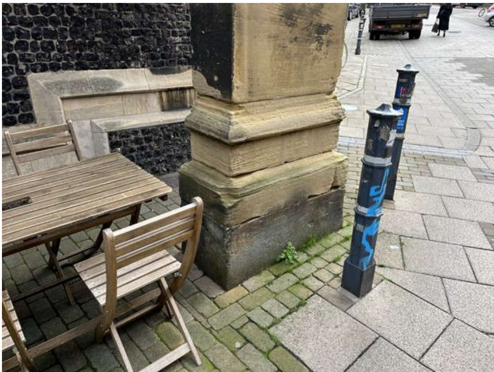
Photograph 14 – Eroded stonework to base of West gable buttresses
