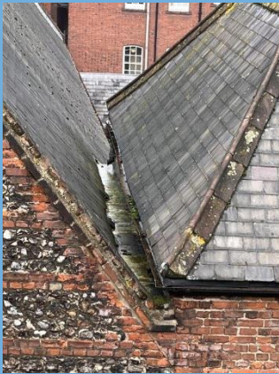
Cloister valley gutter
