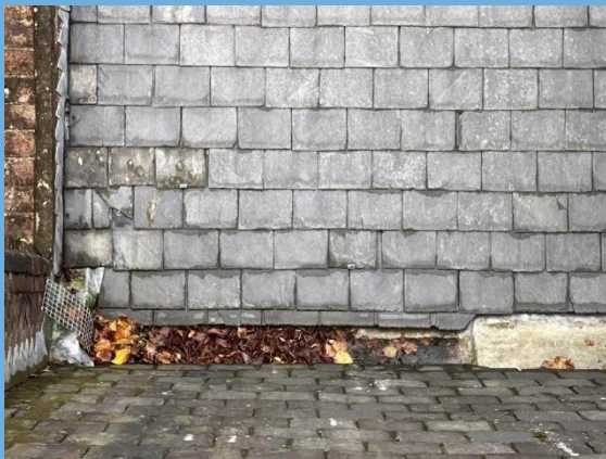
Leaf debris to Cloister valley gutter
