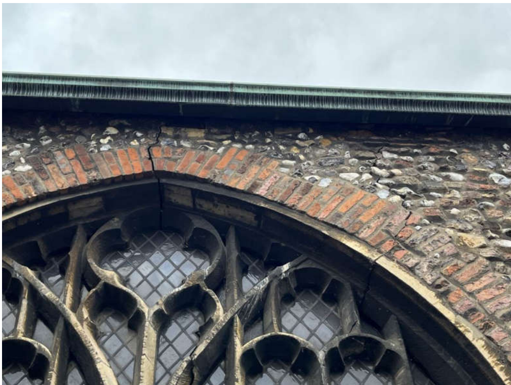
Photograph 8 – Cracking over window arch (western window on North Elevation)
