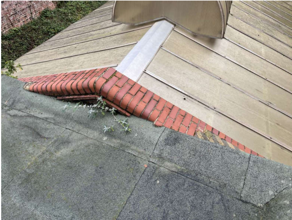
Photograph 85 – No flashing where West gable meets adjacent roof
