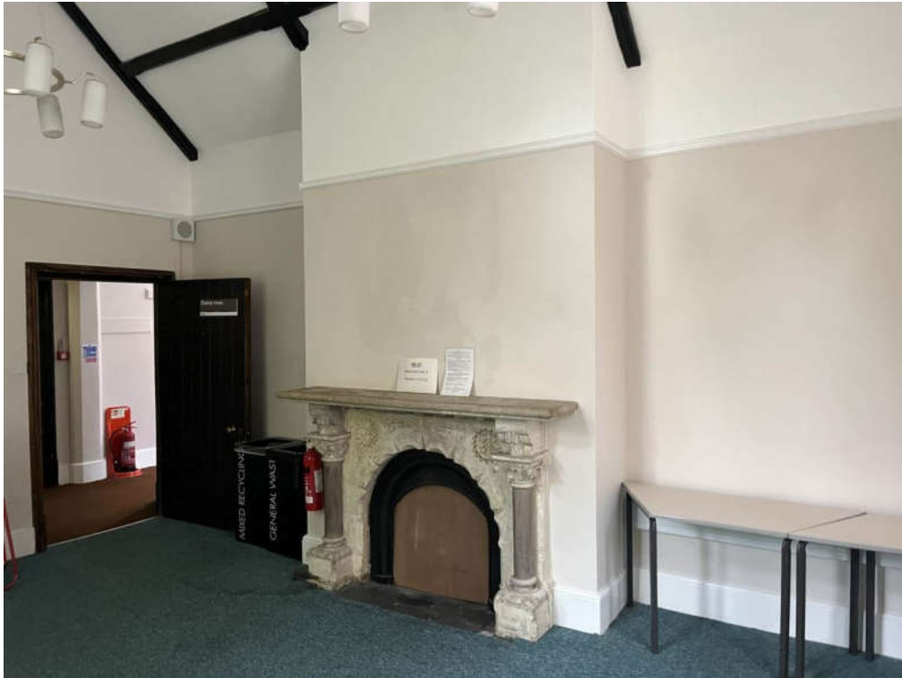
Photograph 73 – Fireplace blocked and signs of damp on chimney breast
