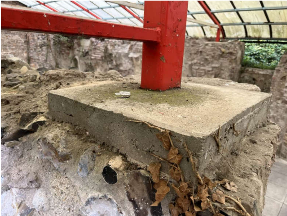
Photograph 91 – Steelwork embedded in concrete pad cast onto wall
