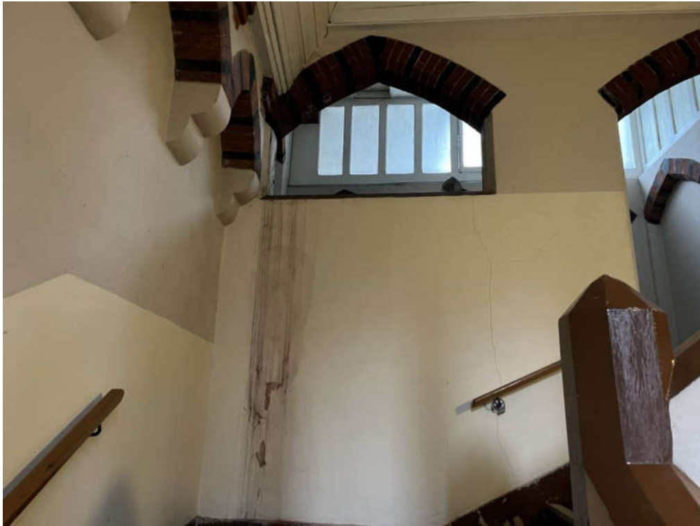
Photograph 75 – Extensive water ingress through roof structure over staircase
