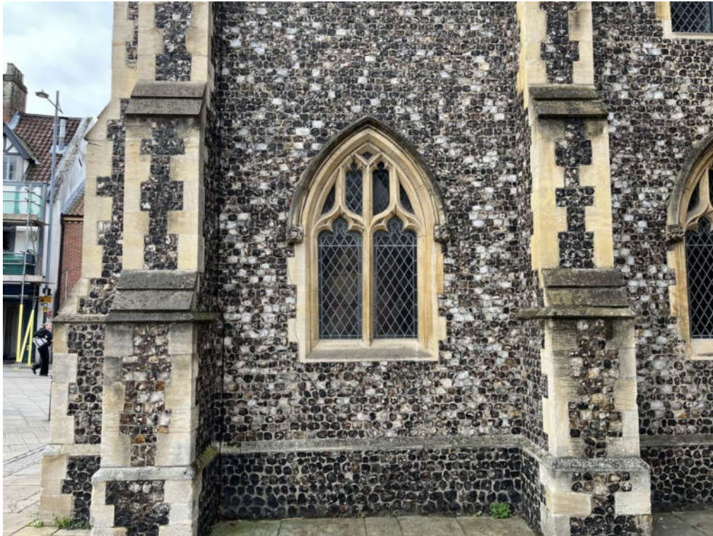
Photograph 11 – Vertical crack below and above South porch window
