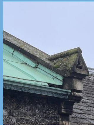
Failed copper flashing to gable
