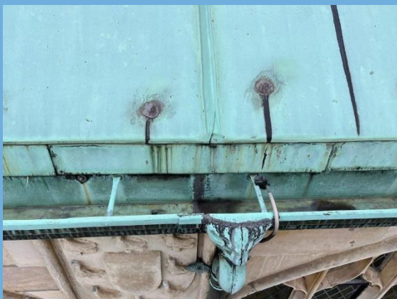
Poor lead fixings to centre of copper sheet
