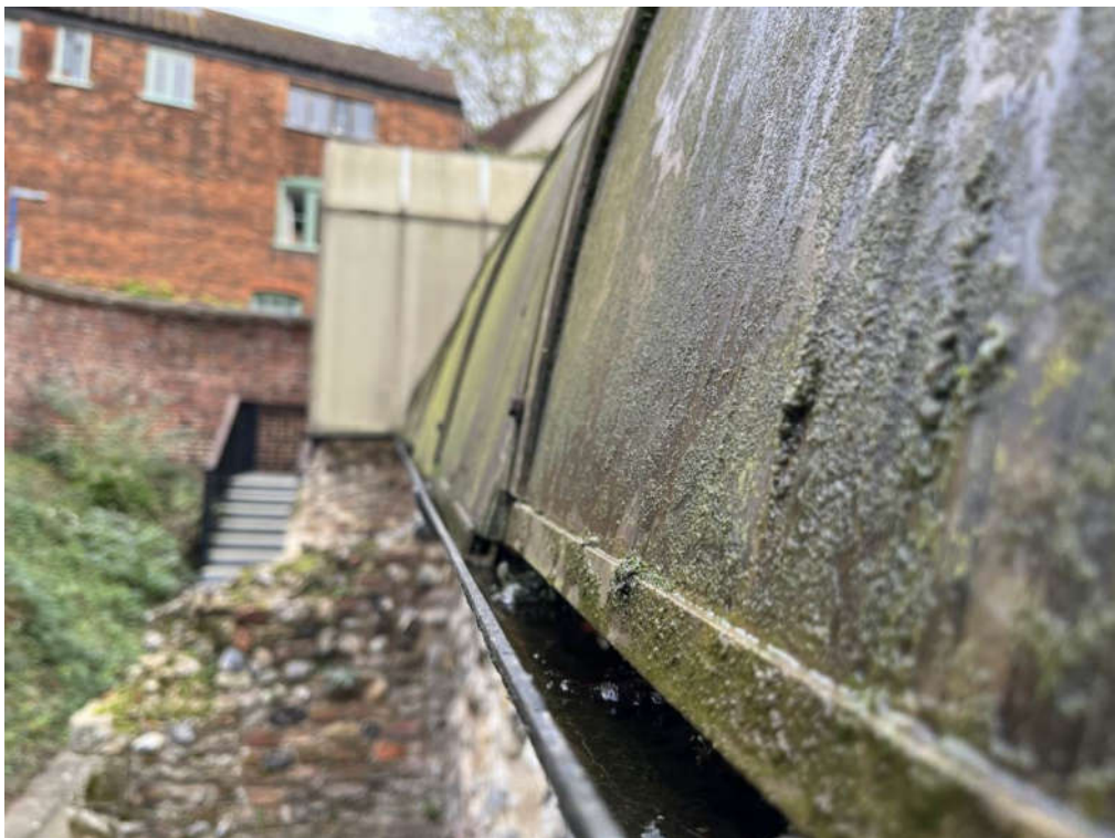
Photograph 88 – Dropped roof sheet and blocked gutters
