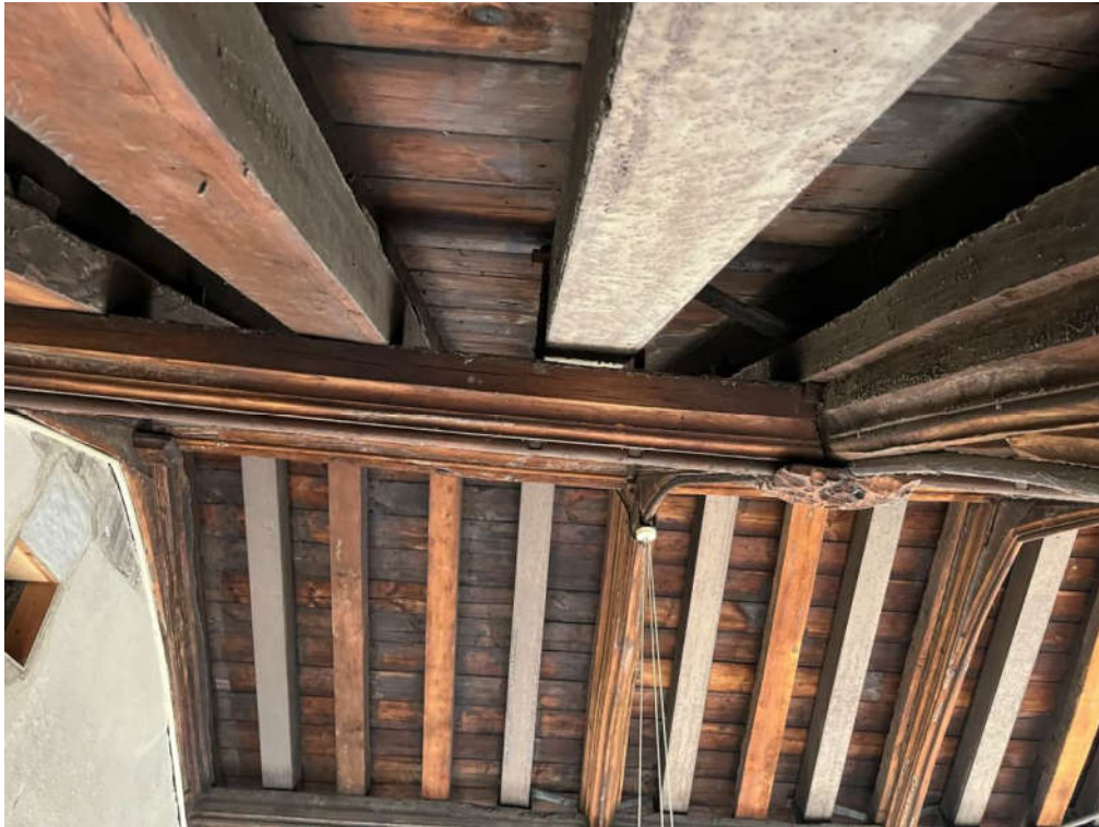
Photograph 41 – Bracket behind rafters assumed to support historic timber truss from new steel trusses either side
