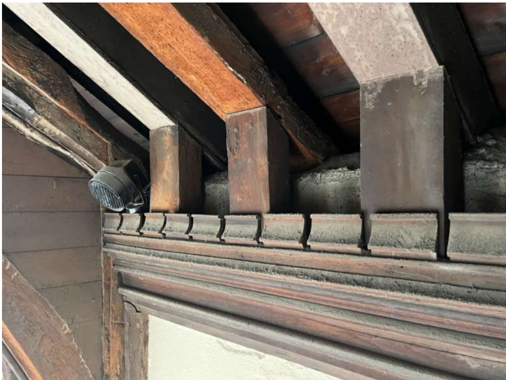
Photograph 42 – Typical eaves detail (concrete eaves beam/infill present)
