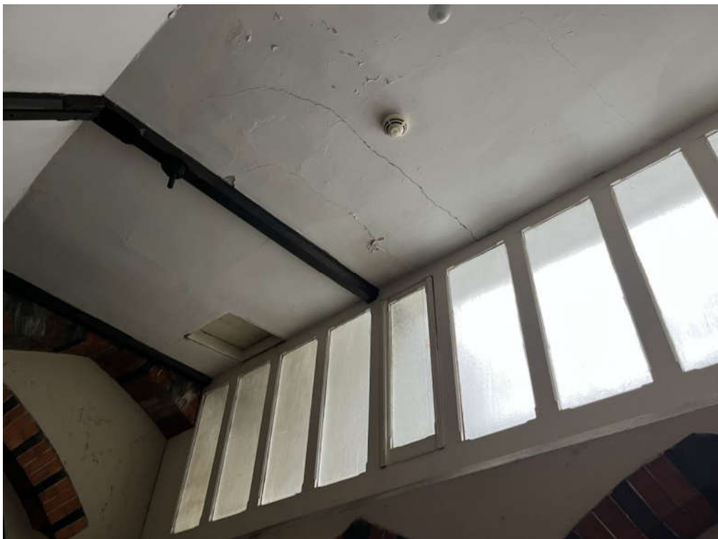
Photograph 76 – Cracking present in ceiling plaster
