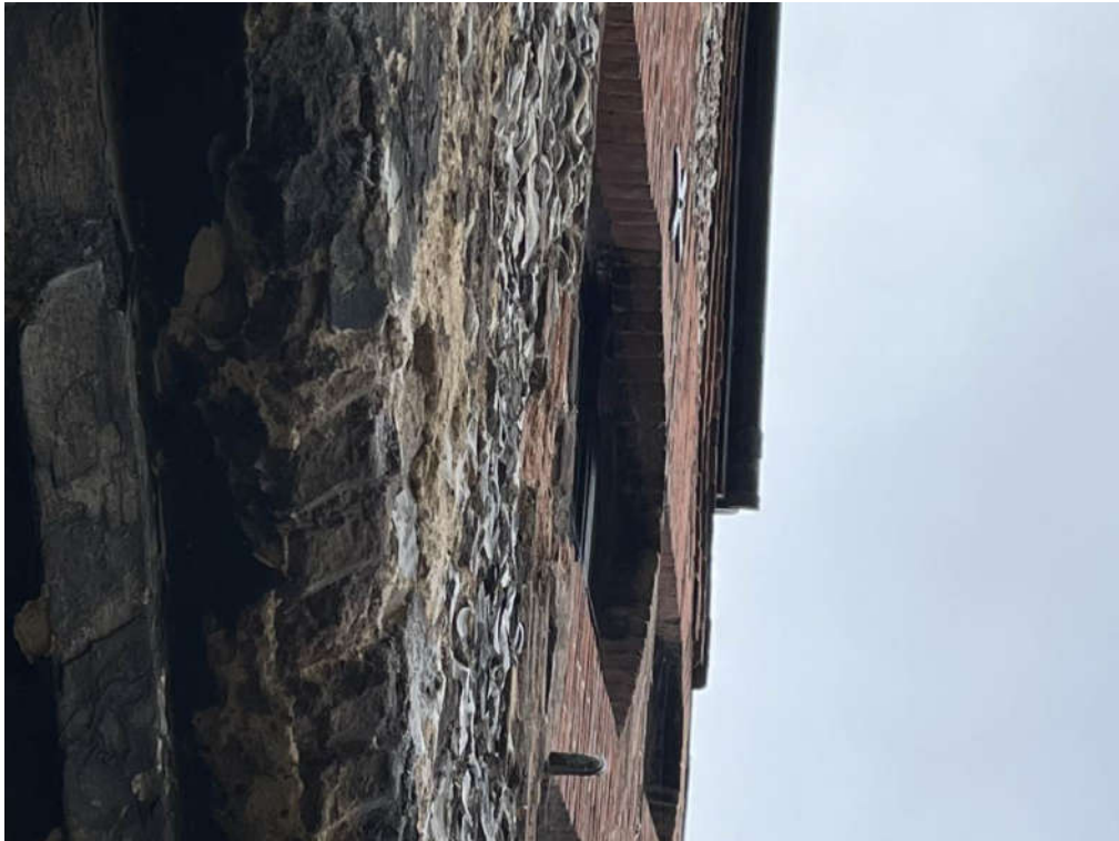
Photograph 53 – Brick window arch bowing out
