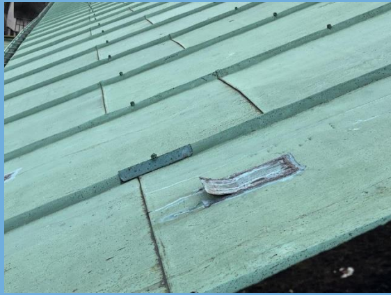
Failed patch repair to copper
