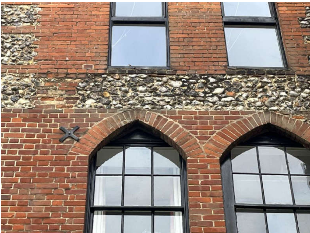
Photograph 54 – Bowed and cracking window arch brickwork
