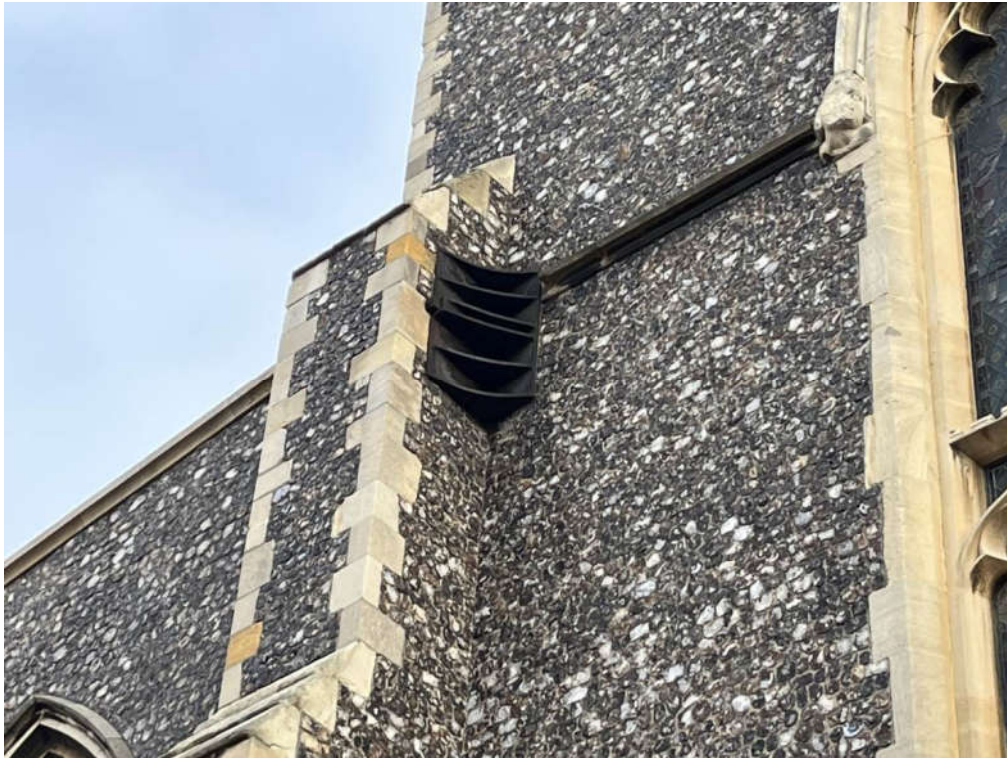
Photograph 15 – Large metal bracket tying West gable construction to end buttresses
