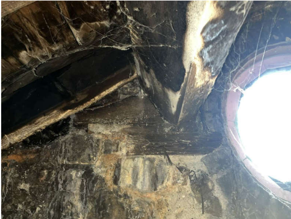
Photograph 31 – Damp timber elements where North purlin extends into East wall (organ loft)
