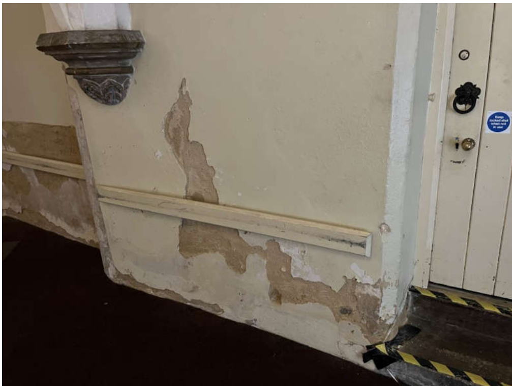
Photograph 62 – Signs of damp in Ground Floor walls
