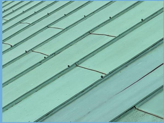
Fixings to copper sheet seams
