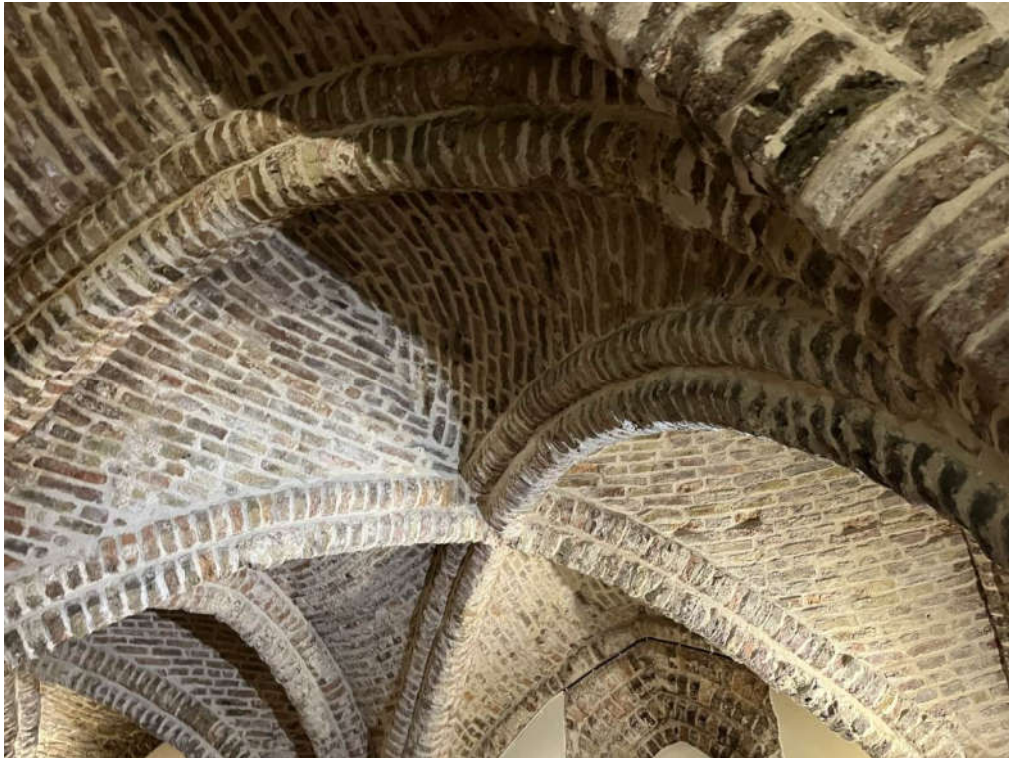
Photograph 79 – Masonry arches repointed in the last century
