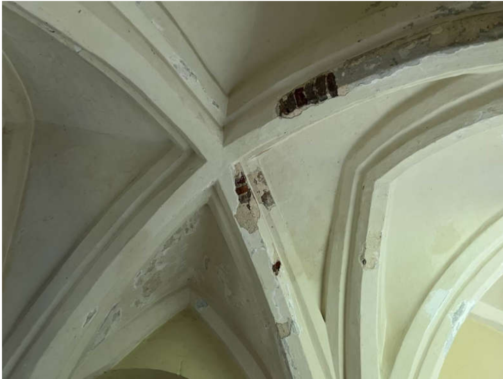
Photograph 61 – Brickwork deteriorated where plaster has fallen away
