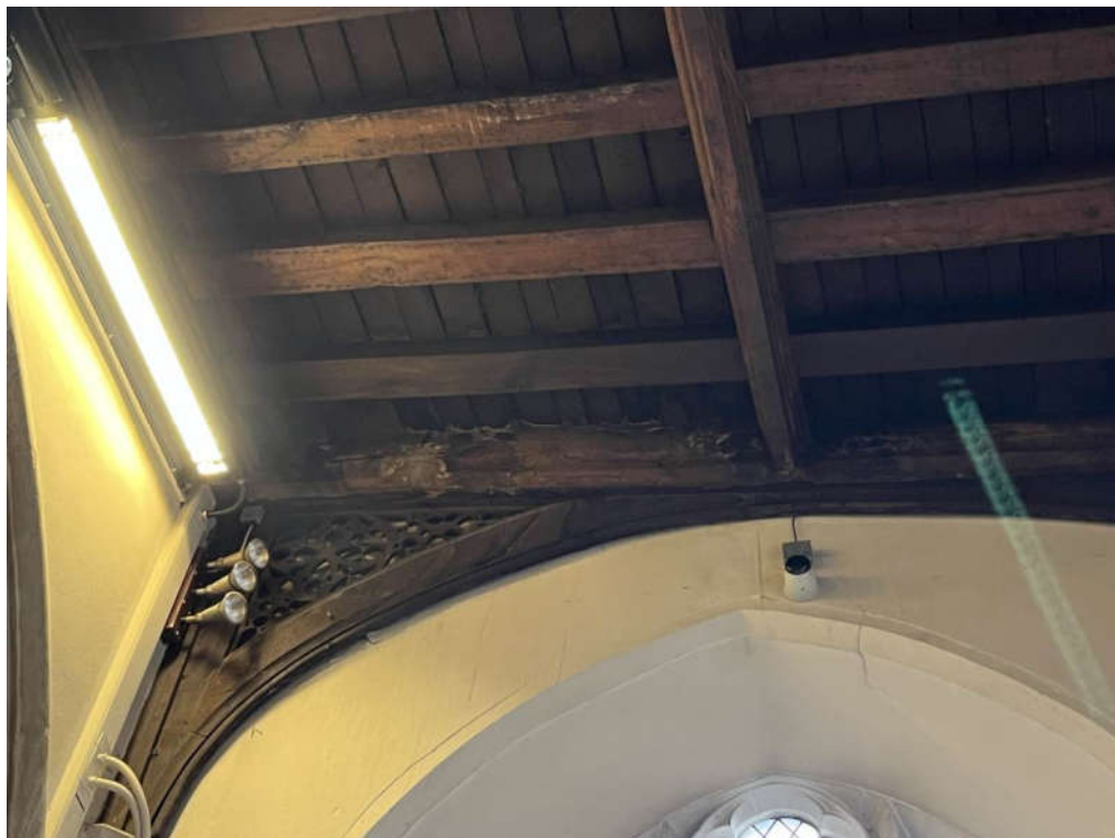
Photograph 24 – Signs of historic damp to East end of South aisle roof structure
