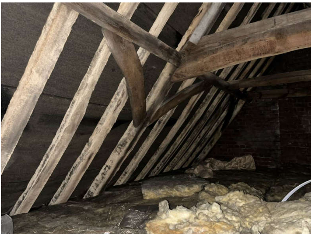
Photograph 68 – In plane bracing
