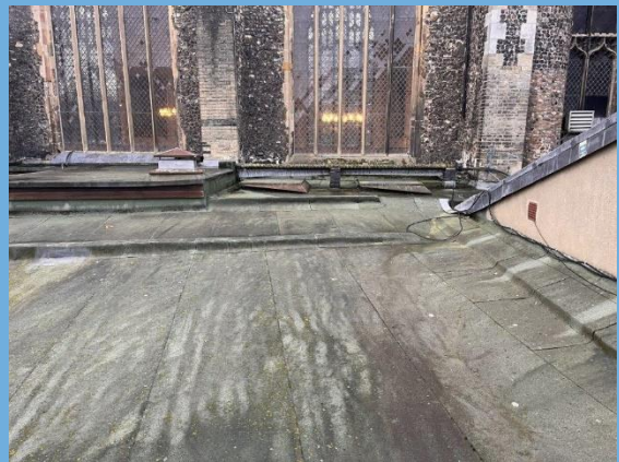
Felt roof in poor condition
