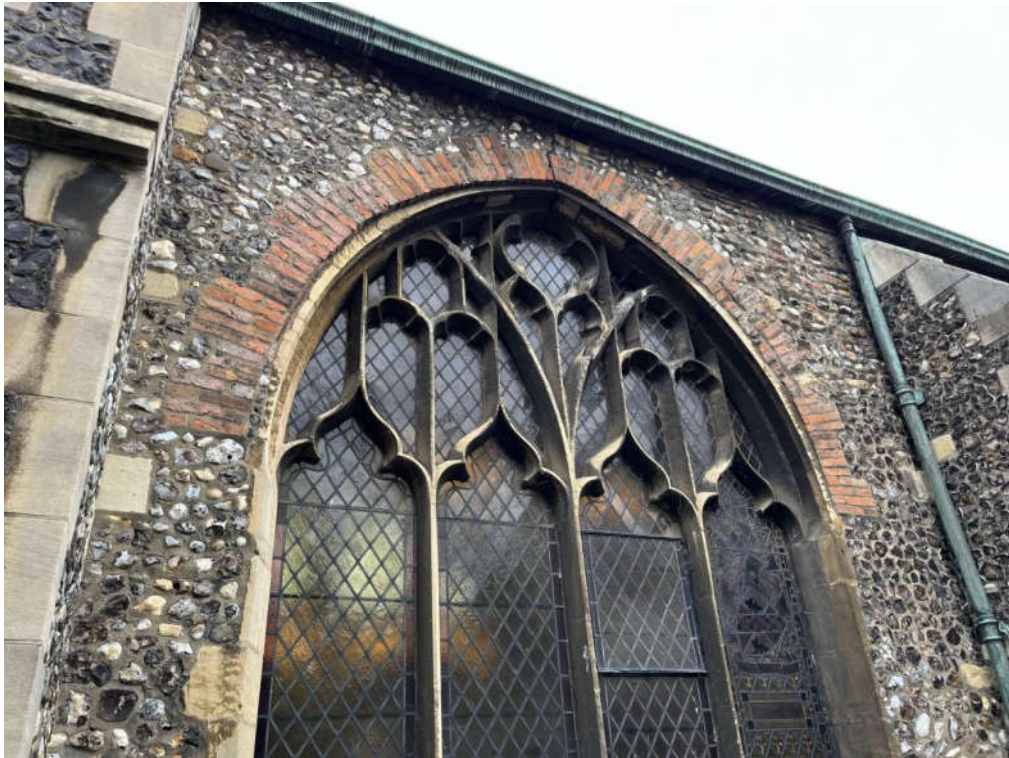
Photograph 9 – Brickwork exposed around North Elevation arches
