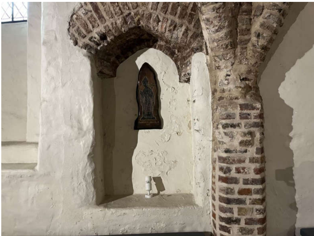
Photograph 82 – Signs of damp in walls
