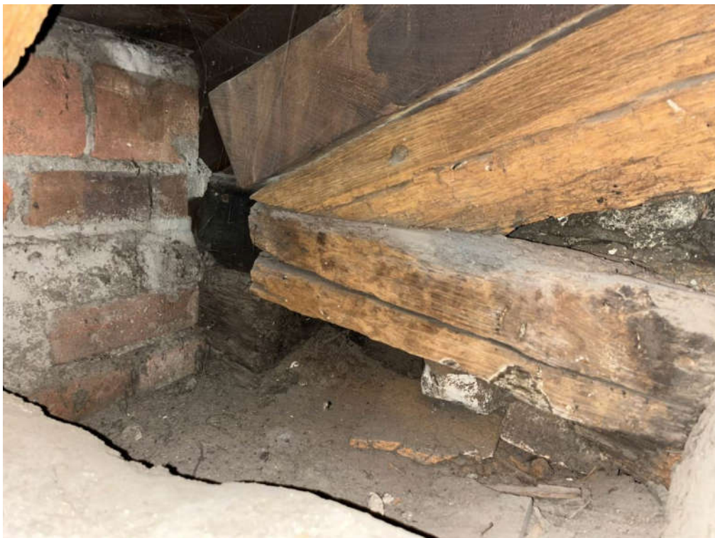
Photograph 28 – Signs of decayed timber at eaves level (common rafter end and plate)
