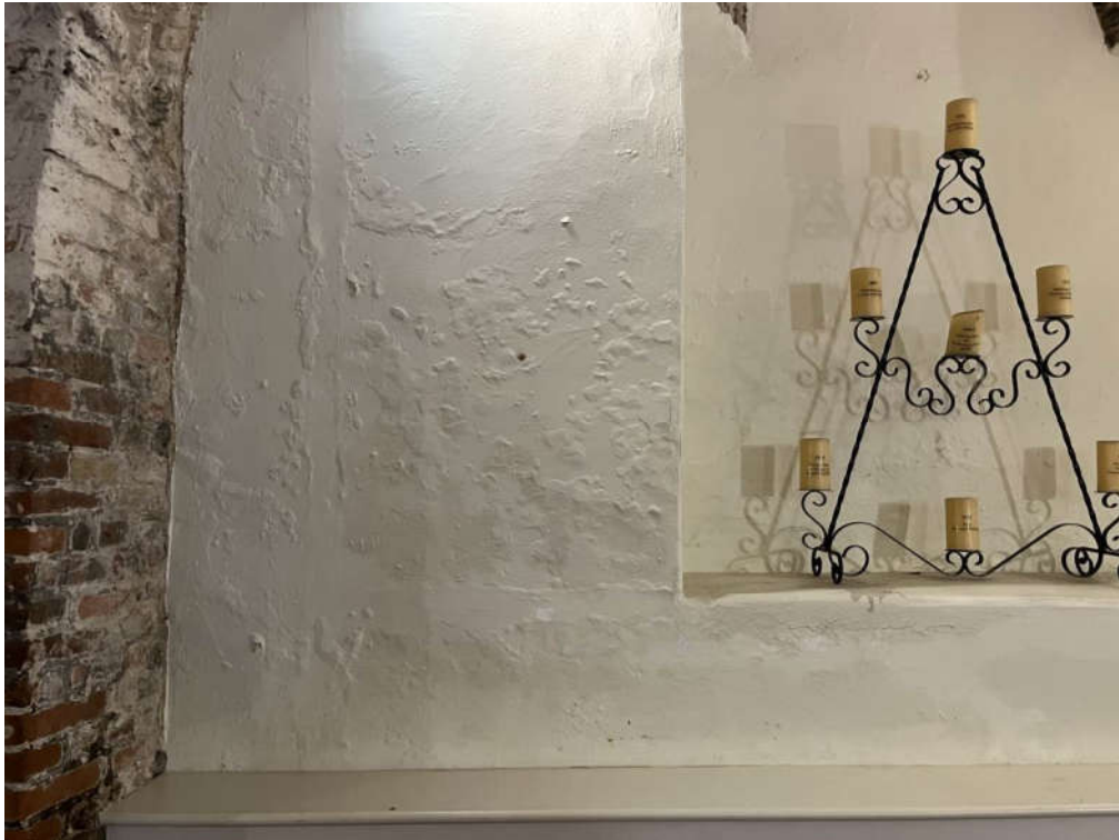
Photograph 81 – Signs of damp in walls
