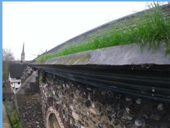
Blackfriars gutter in disrepair
