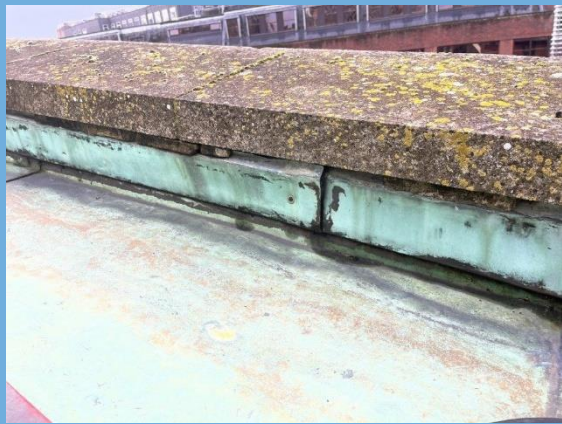
Copper abutments in poor condition
