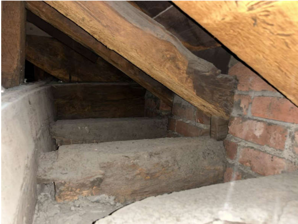
Photograph 27 – Typical common rafter support detail
