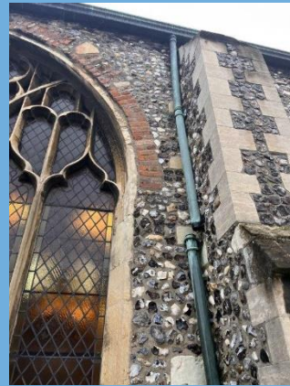
Copper RWG in poor condition
