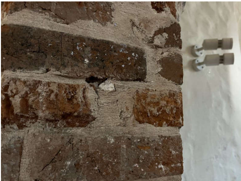
Photograph 80 – Masonry repointed with a hard mortar
