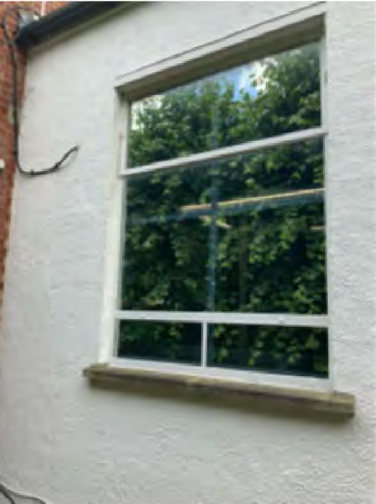
STYLE OF WINDOW TO BE RECOVERED AND REPLACED WITH AN ACOUSTIC LOUVRE FROM THE SINGLE STOREY PART OF THE BUILDING
