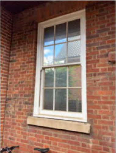
STYLE OF WINDOW TO BE RECOVERED AND REPLACED WITH AN ACOUSTIC LOUVRE FROM THE TWO STOREY PART OF THE BUILDING
