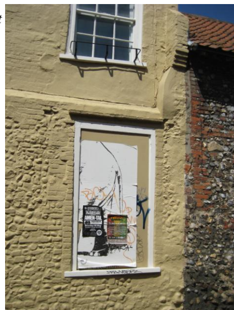
Detail view of boarded sash window to G02.
