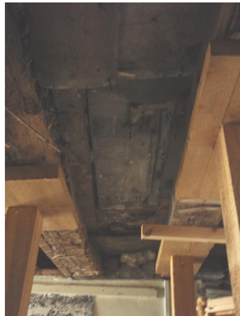
View of temporary props within Gatekeeper's.
