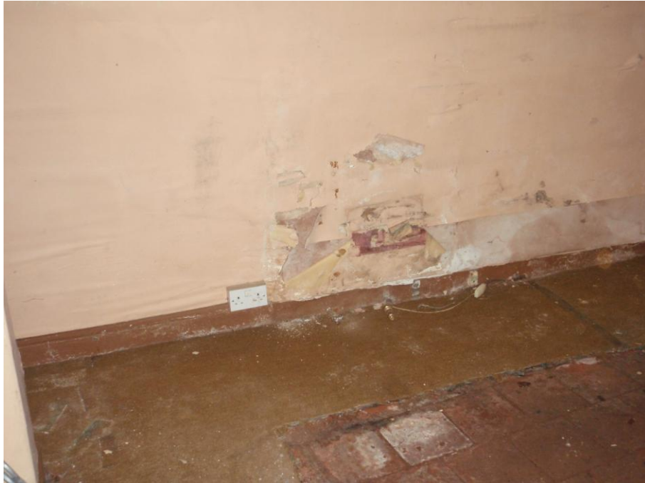
View of proposed utility (G05), showing damp to west wall where external ground levels are 1m above internal finished floor level. Works to improve conditions are described below (see 6.7.1).
