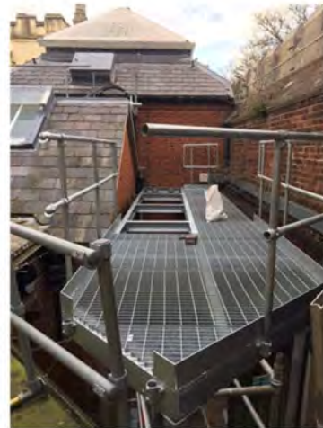
Steelwork Gantry Installed
