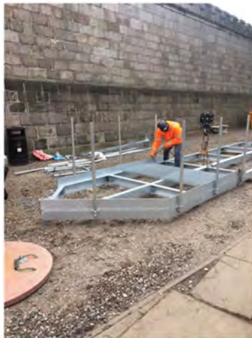
Steelwork Gantry construction
