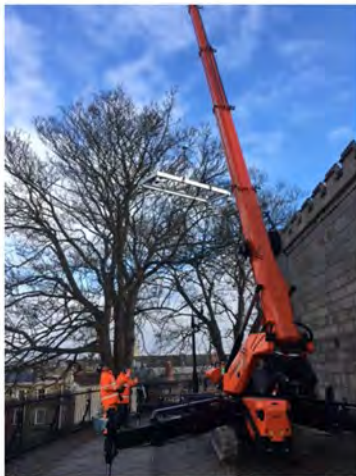
Packing room steelwork Lift
