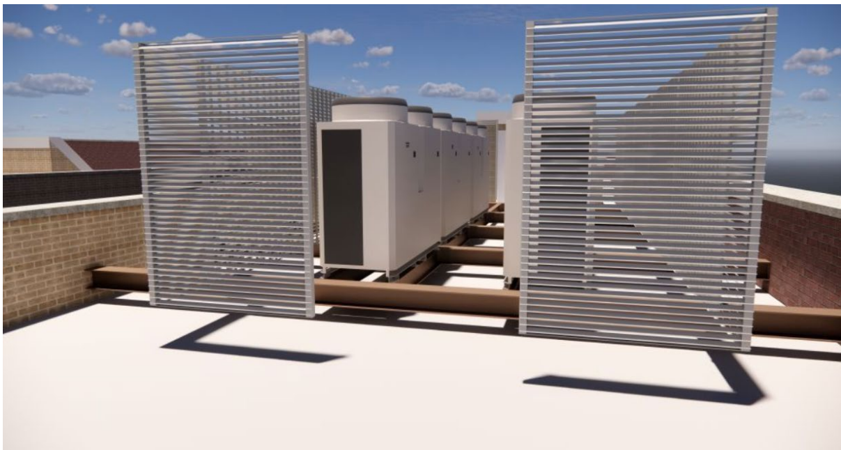
Image 2) Suspended steel structure to allow ASHP install on City Hall Roof.
