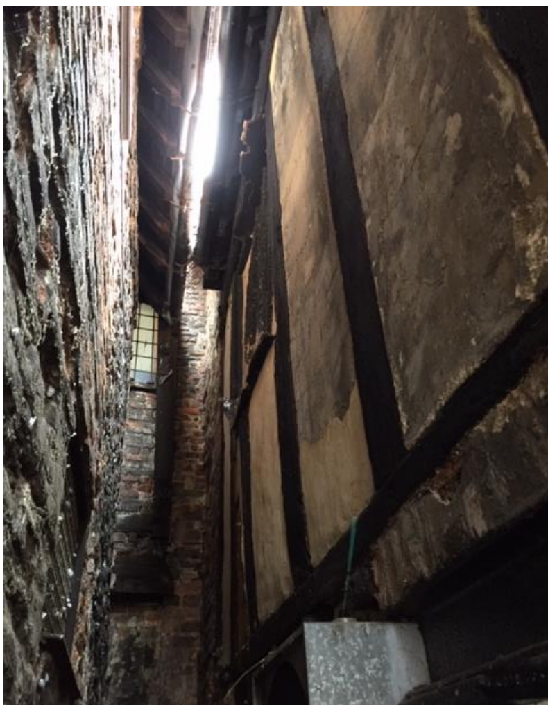
Photo 2 – On right of picture – Timber framed east elevation of the Stranger's Club with the unauthorised extract unit (fire risk) located directly below the C16th timber framed jetty beam. On left of picture - West elevation of 26-28 Elm Hill severely damaged by years of moist fatty flammable emissions in the enclosed gap between the buildings.
