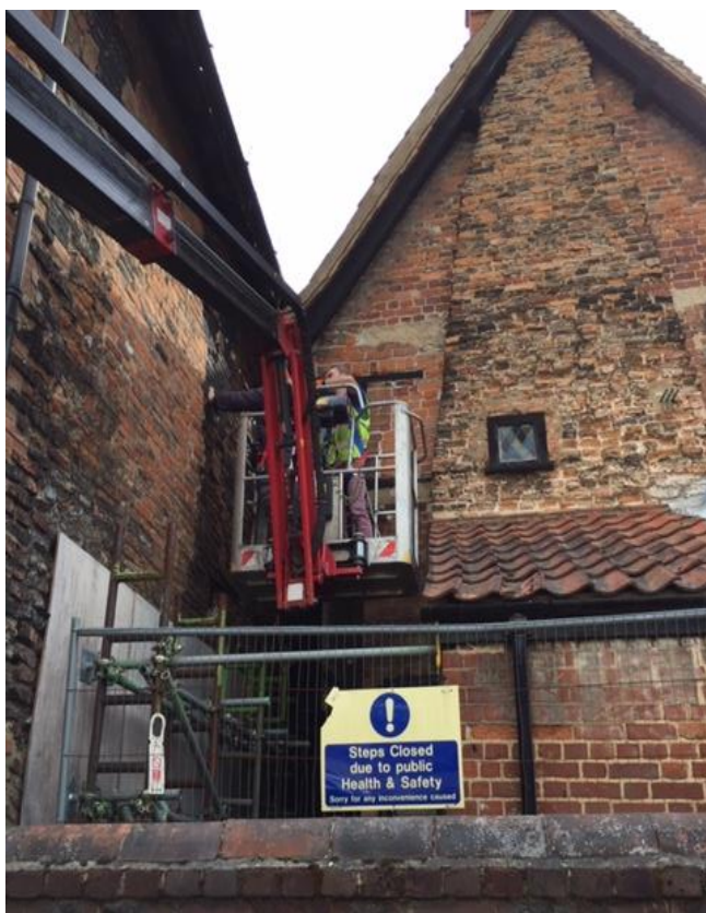
Photo 1 - North elevation (looking from River) of 22-24 Elm Hill (right building) and 26-28 Elm Hill (left building) – showing the extremely narrow gap between the two buildings (into which the flue was unlawfully inserted) and the damaged and structurally compromised west wall of No.26-28.
