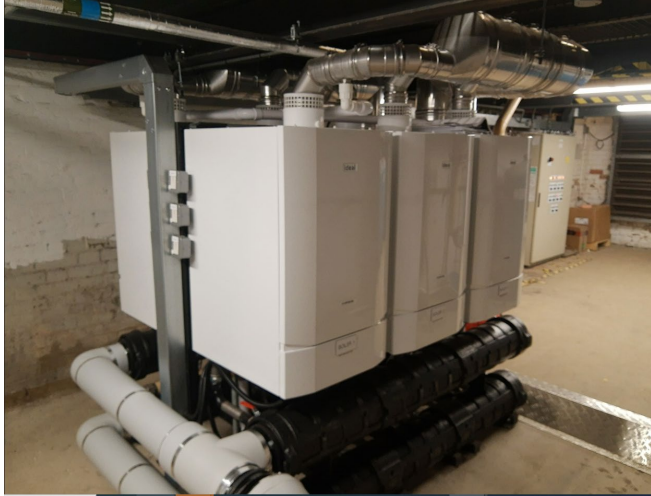
The bank of six new gas boilers following installation
