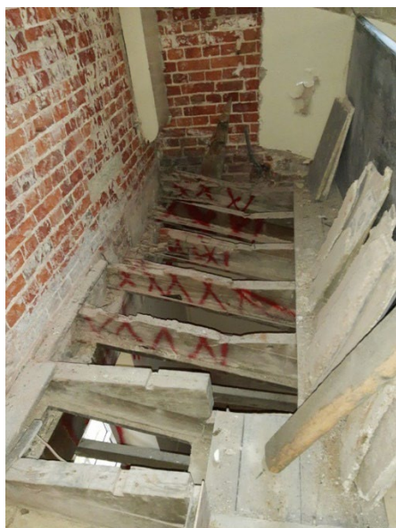
Some of the affected structural timbers
