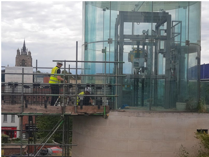
The replacement glazing panel being fixed into place
