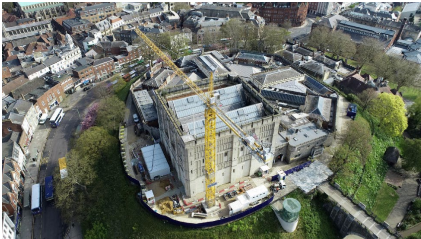
Drone image of the construction site
