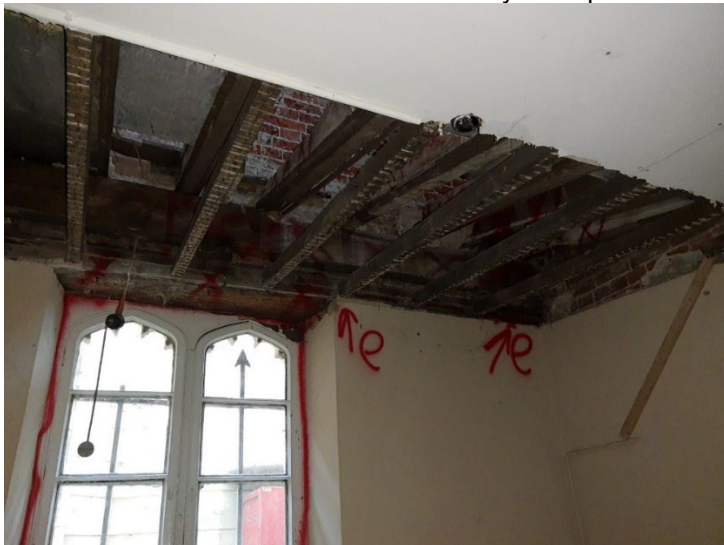
Affected structural timbers beneath the raised seating area
