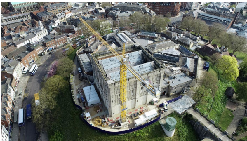
Drone image of the construction site
