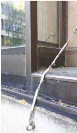
Fig 6.42 Existing windows and the temporary supports required to support the spandrel panels
