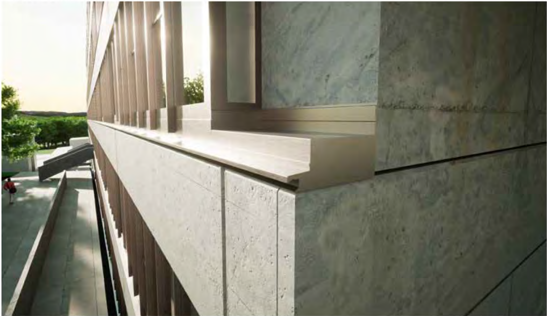
Fig 6.44 CGI of proposed cill detail
