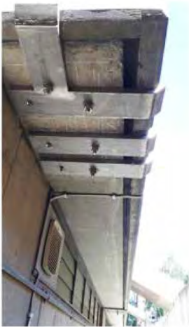
Fig 6.42 Existing windows and the temporary supports required to support the spandrel panels
