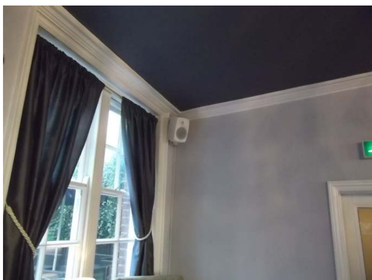
Figure 1: Wall mounted Genelec 4020C loudspeaker
