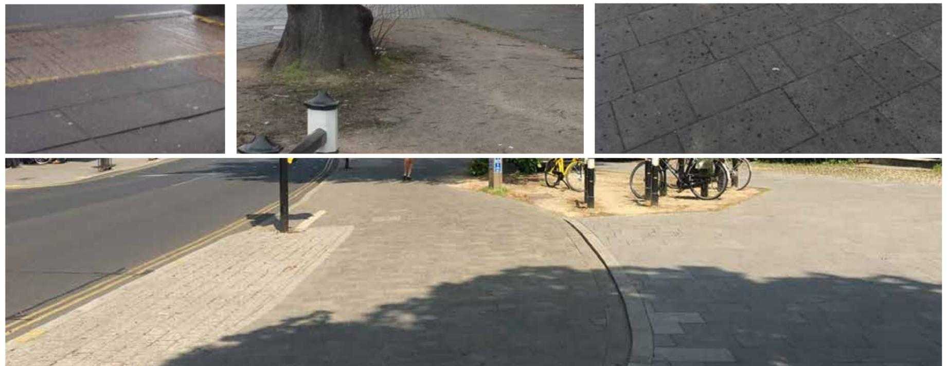
Images clockwise; Concrete paving slabs to pavement with concrete surface to bus stop, hoggin type material around tree, stained paving below tree canopy, new surface types and arrangement to north Tombland.
