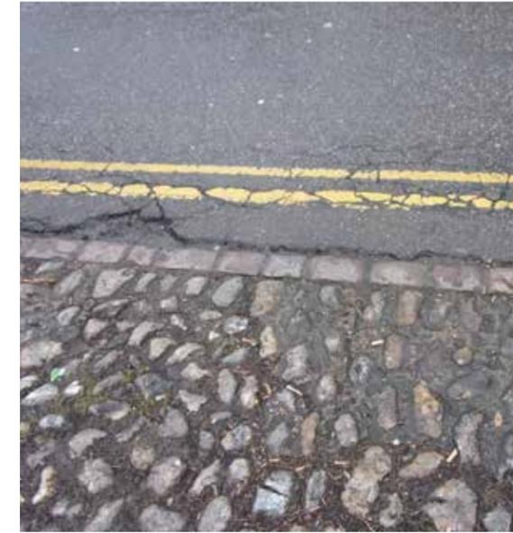
Earth set cobbles with cobble setts to edge of carriageway overlain with Tarmac.
