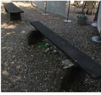
Benches with concrete legs and timber seat. Number of benches in disrepair / with seats missing.
