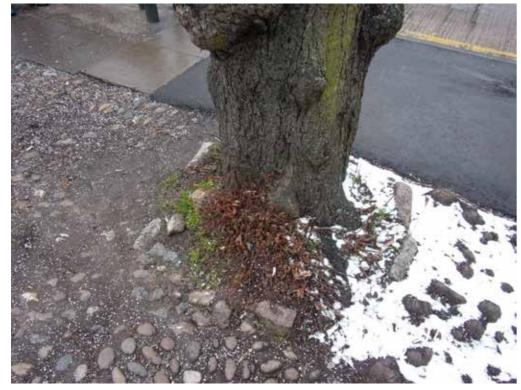
Mixture of materials from different eras. Tree roots lift concrete paving slabs, tarmac replacement temporary solution to root disturbance.
