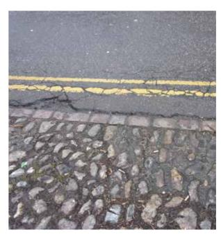
Earth set cobbles with cobble setts to edge of carriageway overlain with Tarmac.
