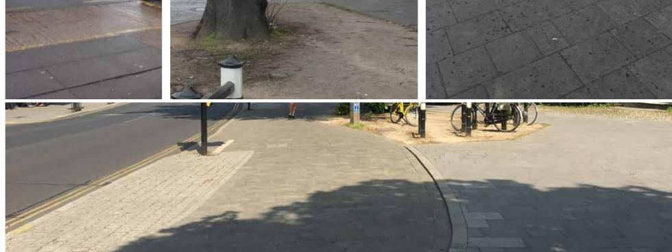
Images clockwise; Concrete paving slabs to pavement with concrete surface to bus stop, hoggin type material around tree, stained paving below tree canopy, new surface types and arrangement to north Tombland.
