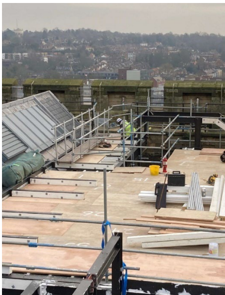
Installation of rooftop platforms on Keep
