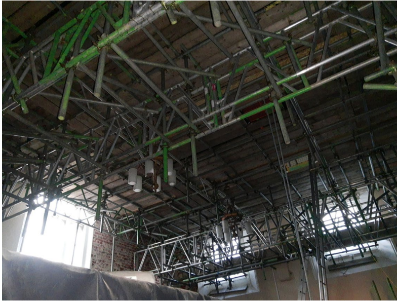
The internal bird nest scaffolding within the Courtroom
