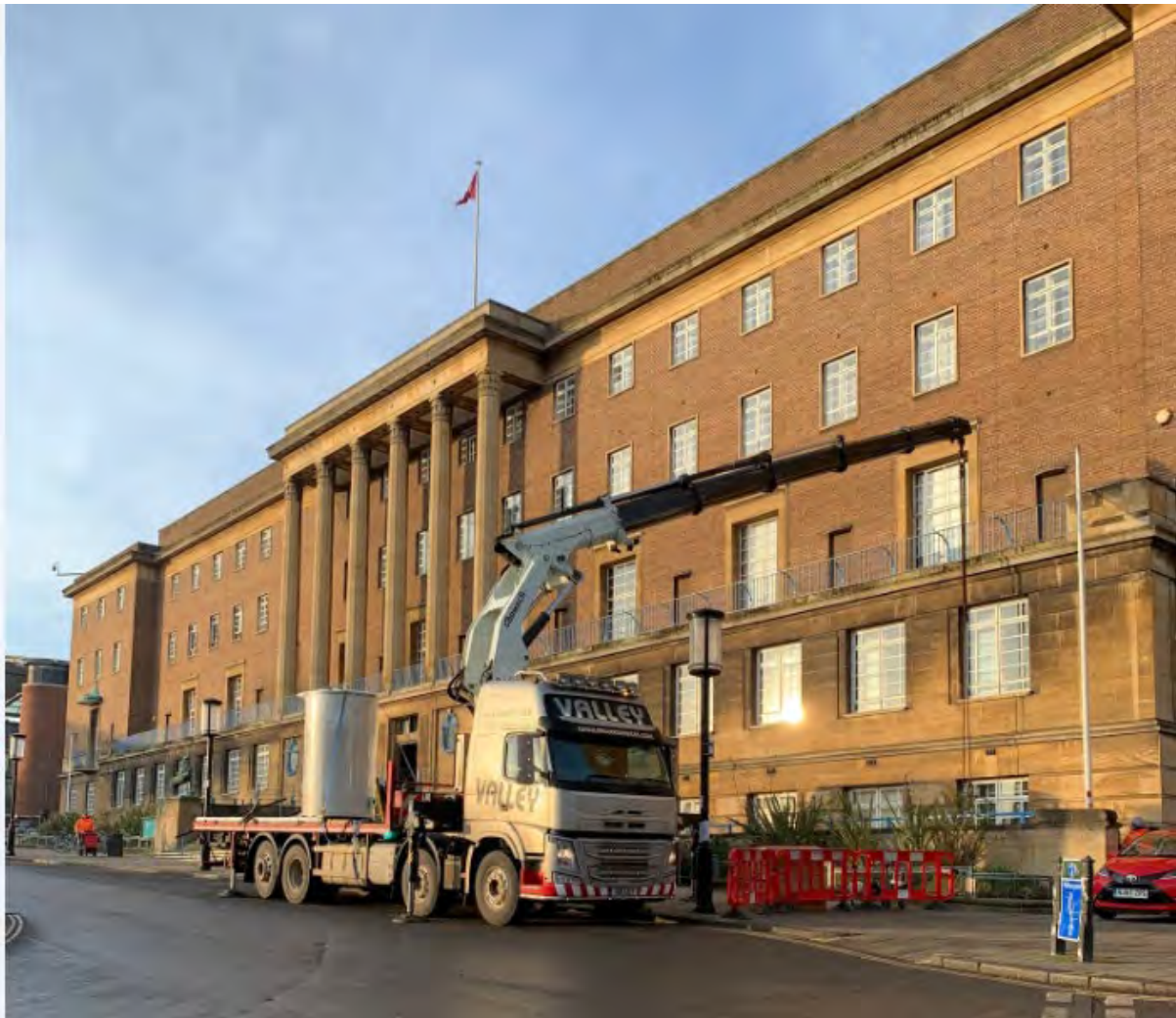
Figure 1 Showing crane lift into City Hall Basement
