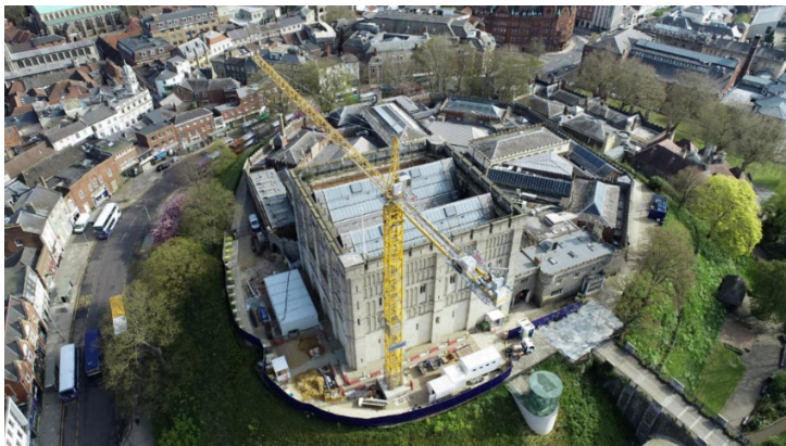
Drone image of the construction site
