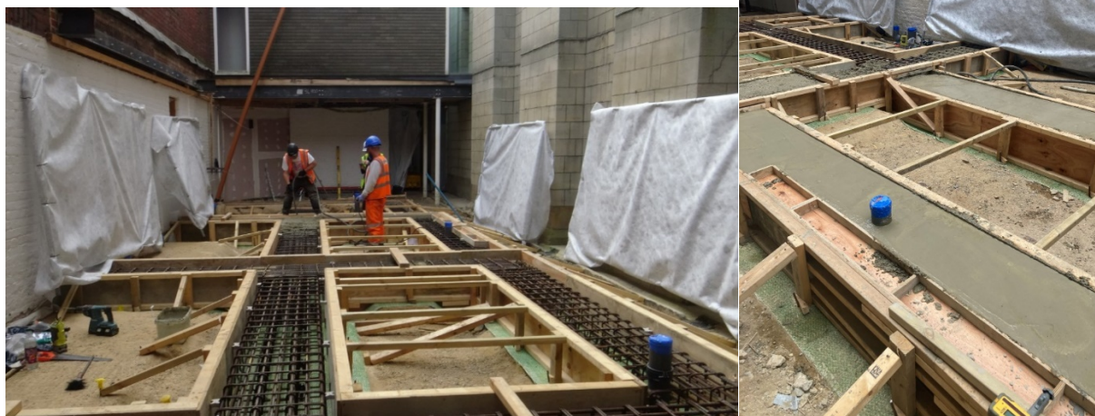
Before and after the pouring of concrete foundations in the new WC block area
