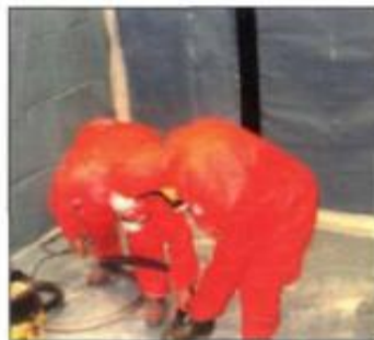
'Buddy' cleaning using a Class H vacuum cleaner
