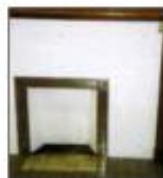
Asbestos insulating board (AIB) fire surround
