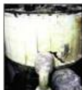
Asbestos lagging on an old tank
