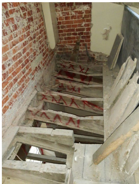
Some of the affected structural timbers
