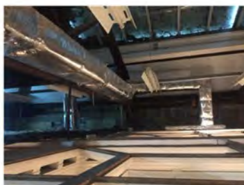
Ductwork Lagged to Scaffolded Areas
