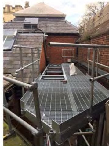
Steelwork Gantry Installed
