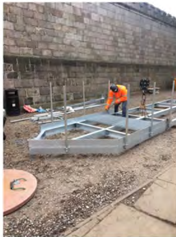
Steelwork Gantry construction
