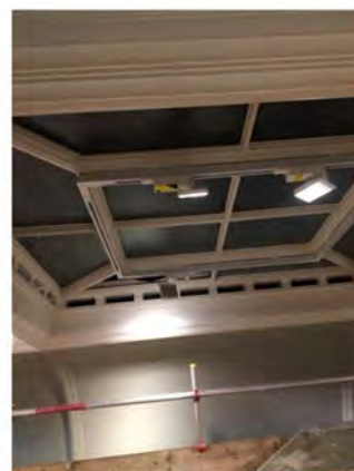
Glazing reinstalled to Norwich Union gallery
